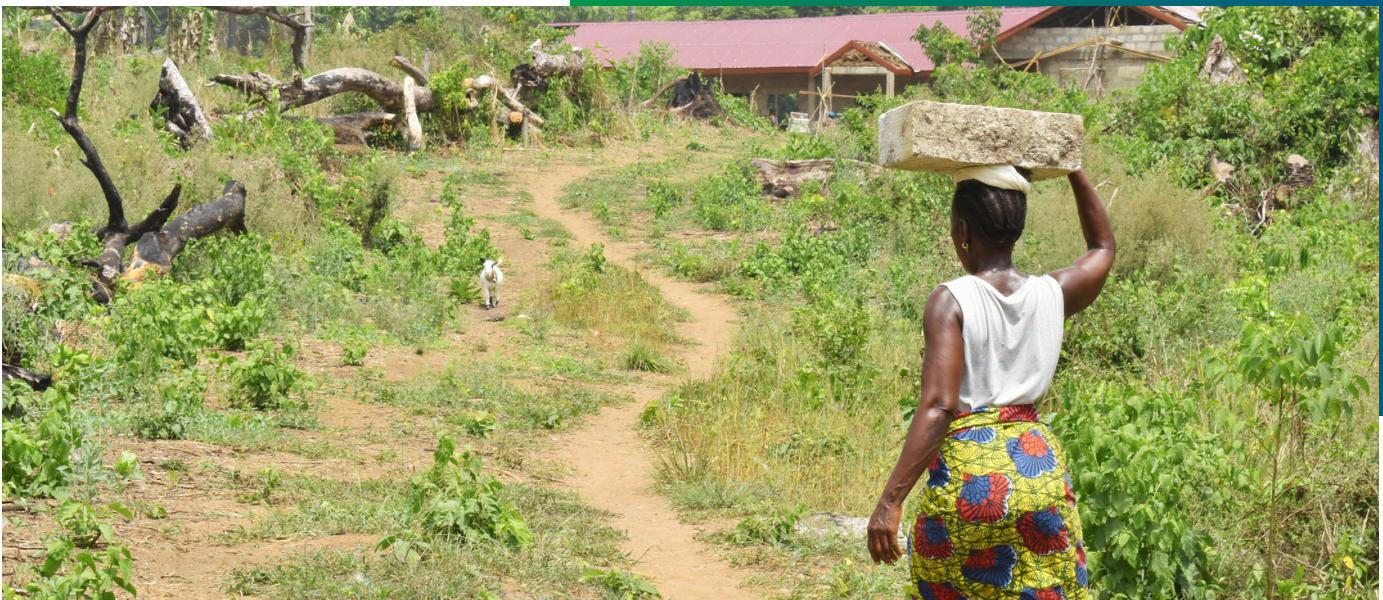
Majoe community member carrying bricks to the community's Lead project site
